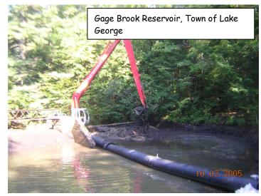
Gage Brook Reservoir still captures a significant amount of sediment and debris on an annual basis (up to 200 cubic yards per year). This reservoir has been the most consistently maintained under this sediment basin program, due to the speed at which it fills with sediment and the relative ease of cleaning it out.
