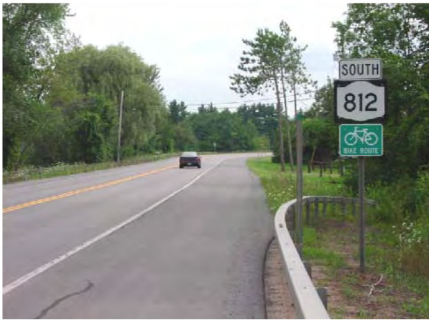
Figure 3 - Bike shoulders (photo courtesy of ANCA)
