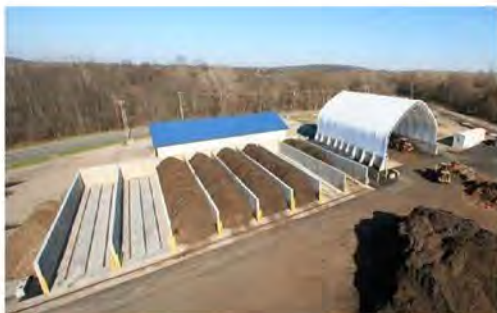
Figure 3-8 Aerated Static Pile Composting
