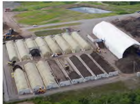
Figure 3-11 Example Covered Aerated Static Pile (C-ASP) Facility
