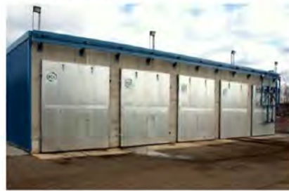
Figure 3-10 Example Containerized In-Vessel Aerated Static Pile
