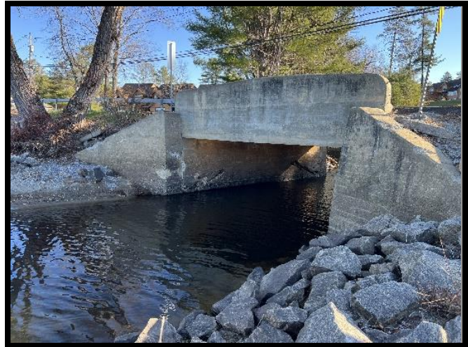
East Shore Drive (CR 15) over Mill Brook (aka Adirondack Bridge)
