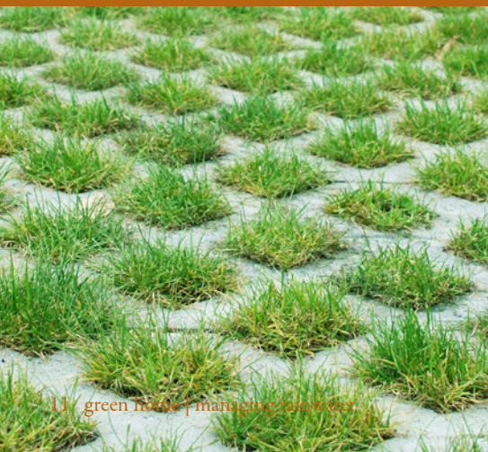
Photo top left: © The Watershed Company. Belgard permeable pavers on a residential patio.
